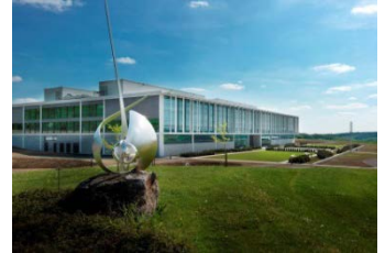
The WITTENSTEIN Innovation Factory is officially opened in May 2014 in Igersheim-Harthausen.
